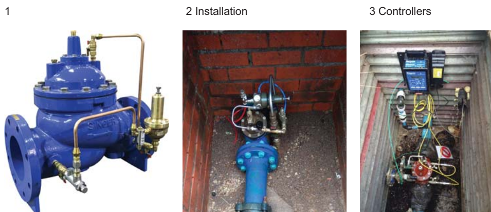
Figure 18 Typical PRV and installation (Sources: Mueller Water Products Inc. (1), K Atkinson (2, 3))
