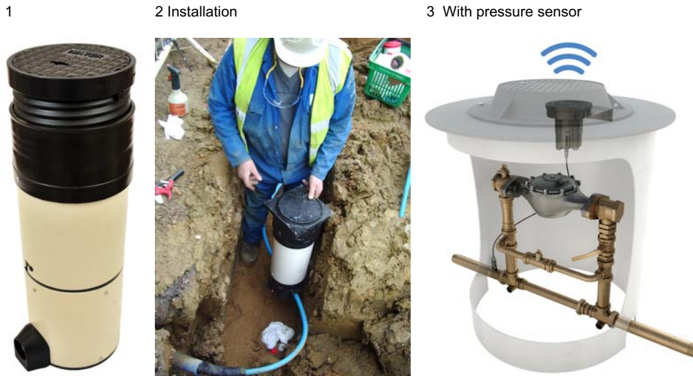
Figure 8 Typical external meter box and Installation (Sources: Plasson (1), J Parker (2), Mueller Water Products Inc. (3)).
