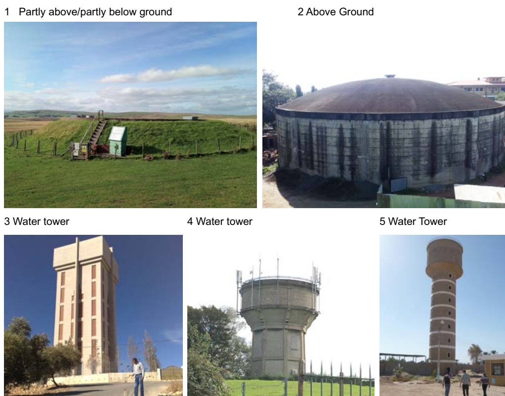
Figure 1 Typical service reservoirs (Sources: K Atkinson (1, 2, 3, 5) and D Pearson (4)).
