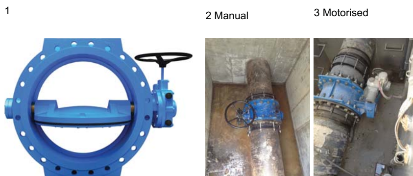
Figure 17 Typical butterfly valves and installation (Sources: Mueller Water Products Inc. (1), K Atkinson (2, 3)).
