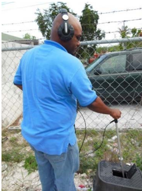
Figure 31 Photograph showing use of electronic listening stick (Source: S Hamilton).
