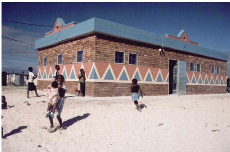
Figure 10.11 Completed chamber in Khayelitsha.
