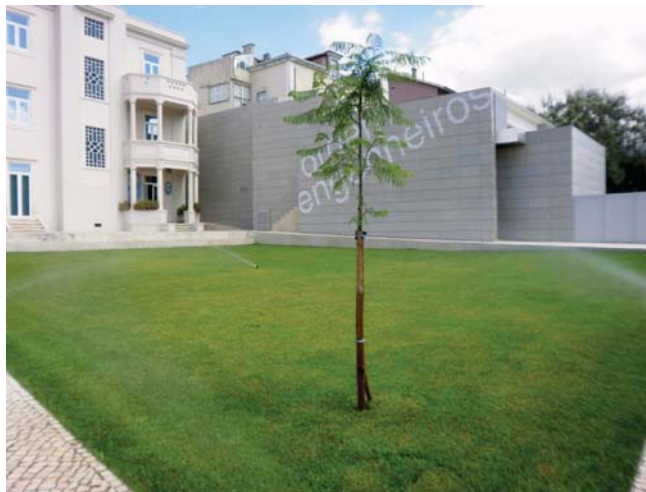
Figure 10.15 The sprinkler system.
