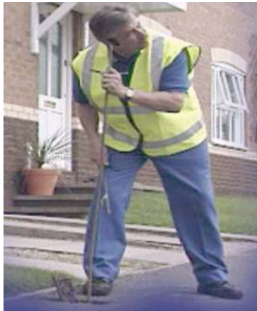
Figure 7: A leakage engineer locating a leak using a traditional listening stick.
