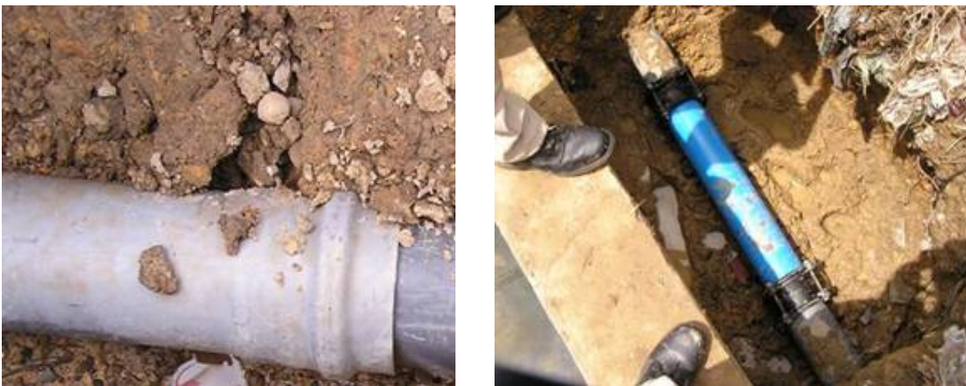
Figure 36: Typical Repair of a leaking Joint
