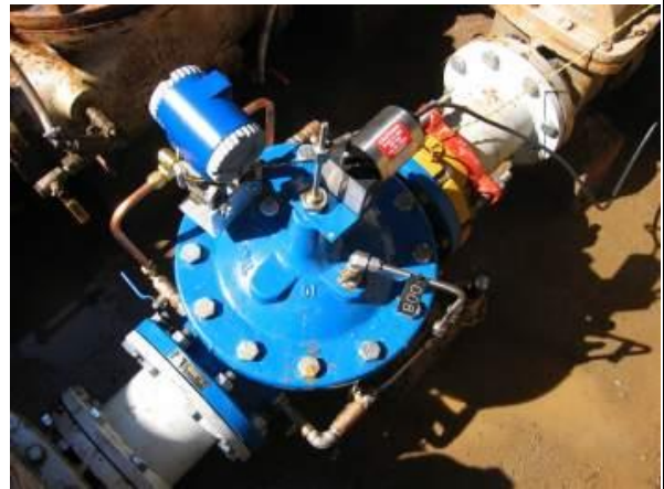
Picture 2: Metering PRV on bypass.
