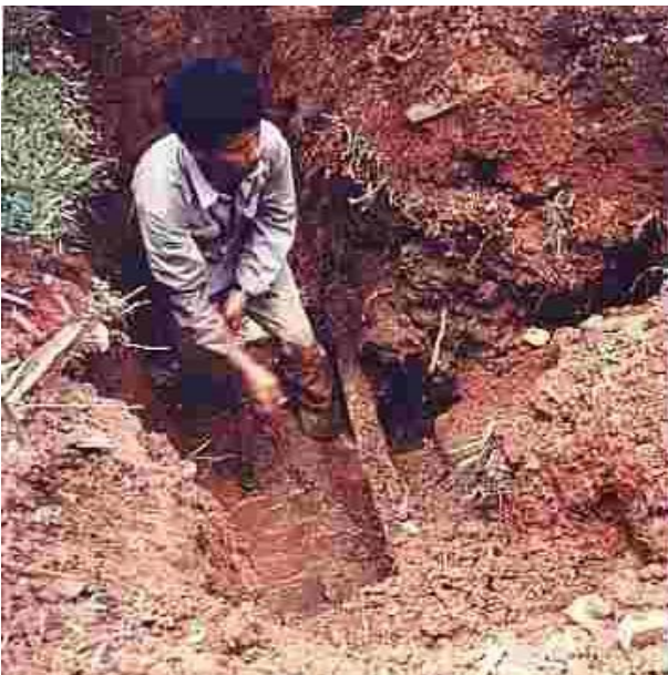
Figure E-2 Excavation by hand.
