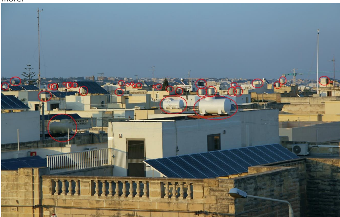
Figure 23 – Properties with roof storage tanks on Malta.
