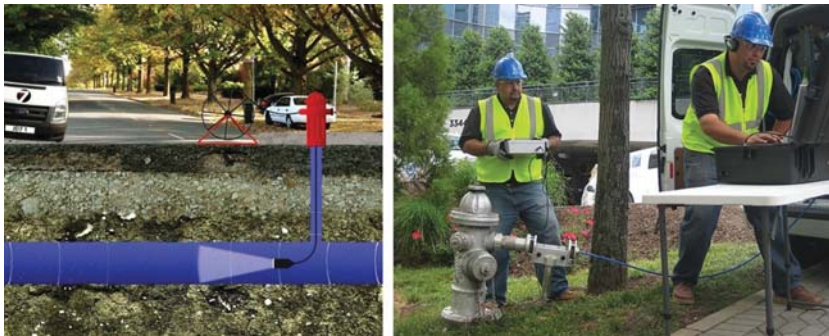
Figure 5.2 Push tethered system which can be operated with or against the water flow with access through tapping point or fire hydrant. (Source: JD7 Ltd)
