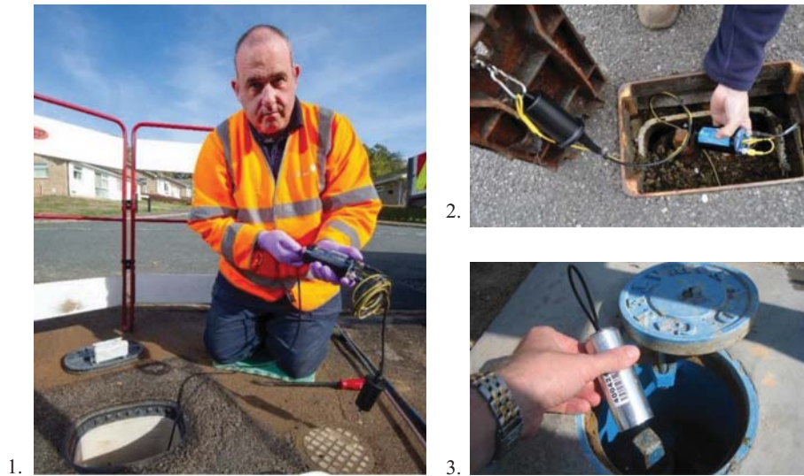
Figure 4.8 Remote correlating logger installation. (Sources: 1 and 2 – Anglian Water/Primayer; 3 – Gutermann)
