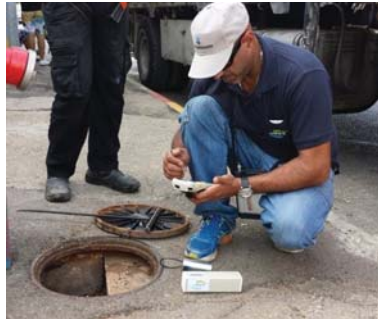
Figure 17.12.4 Mei Carmel staff deploying a correlating logger. (Source: Gutermann)
