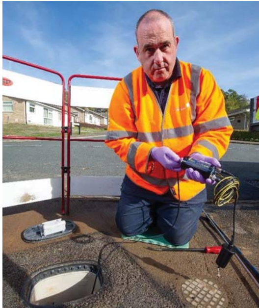
Figure 17.10.1 Installing Enigma3hyQ. (Source: Anglian Water)
