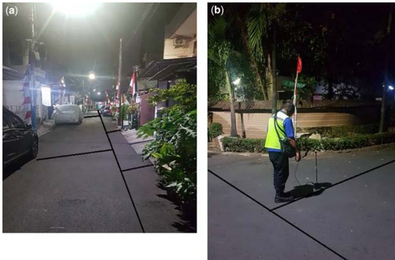
Figure 7.6 (a,b) Checking for leaks at night-time. (Source: Stuart Hamilton).
