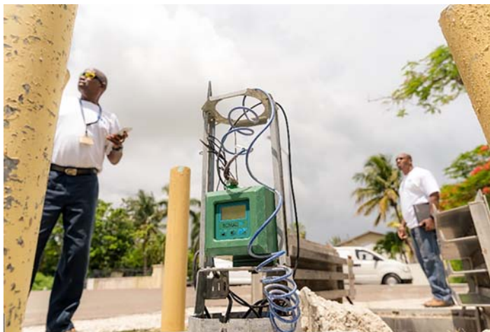
Figure CS2.1 Data loggers gathering system data on flow and pressure (source: Miya Water).
