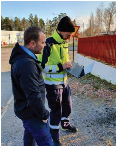
Figure CS6.2 The flow meter data is uploaded to a laptop using the READY programme.
