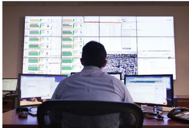
Figure CS10.4 Mueller Network Operation Center (NOC) in Atlanta, Georgia.
