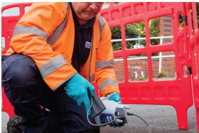
Figure CS3.1 Final installations of the latest NB-IoT (Narrow Band Internet of Things) pilot technology were recently underway (source: Envirotec magazine).
